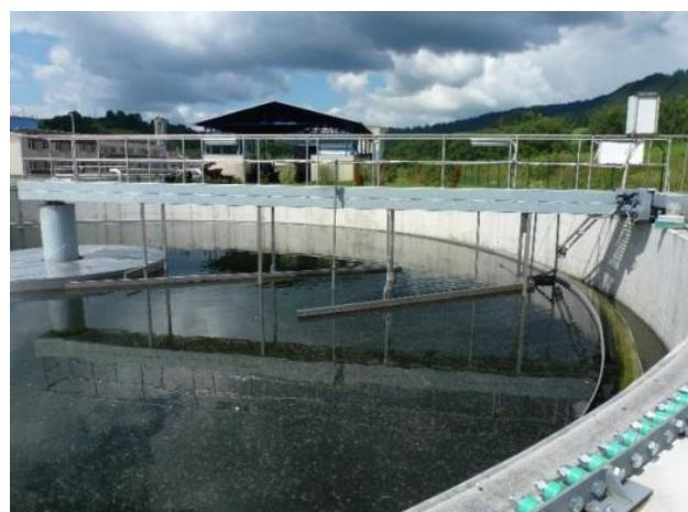
**Figure 2: Radial settling tank
