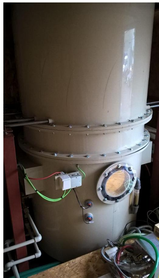
Figure 8B: Body of biotrickling filter
