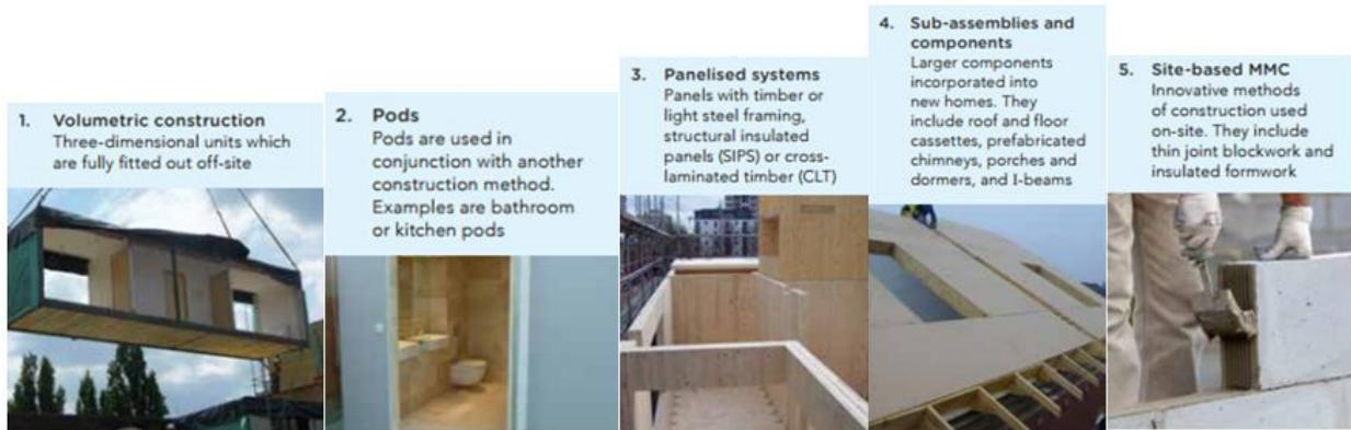
**Figure 1: Types of MMC according the NHBC Foundation<sup>7</sup>**
