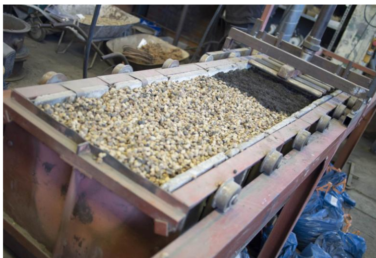
Figure 3: Horizontal sinter grate
