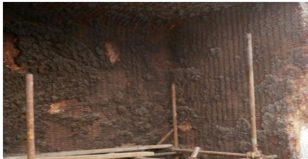
**Figure 1: Deposits on the walls on the entrance in the 1st boiler draft - during reconstruction**
