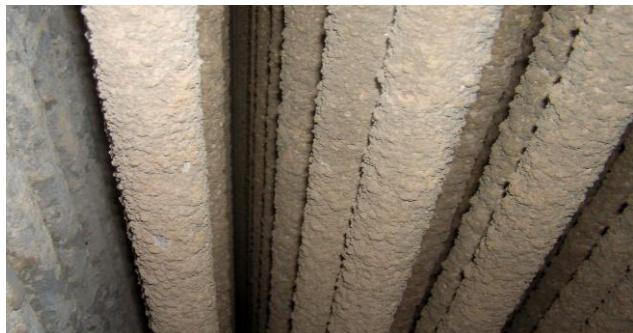
**Figure 2: Deposits on the heat exchange surfaces in the 2nd boiler draft**
